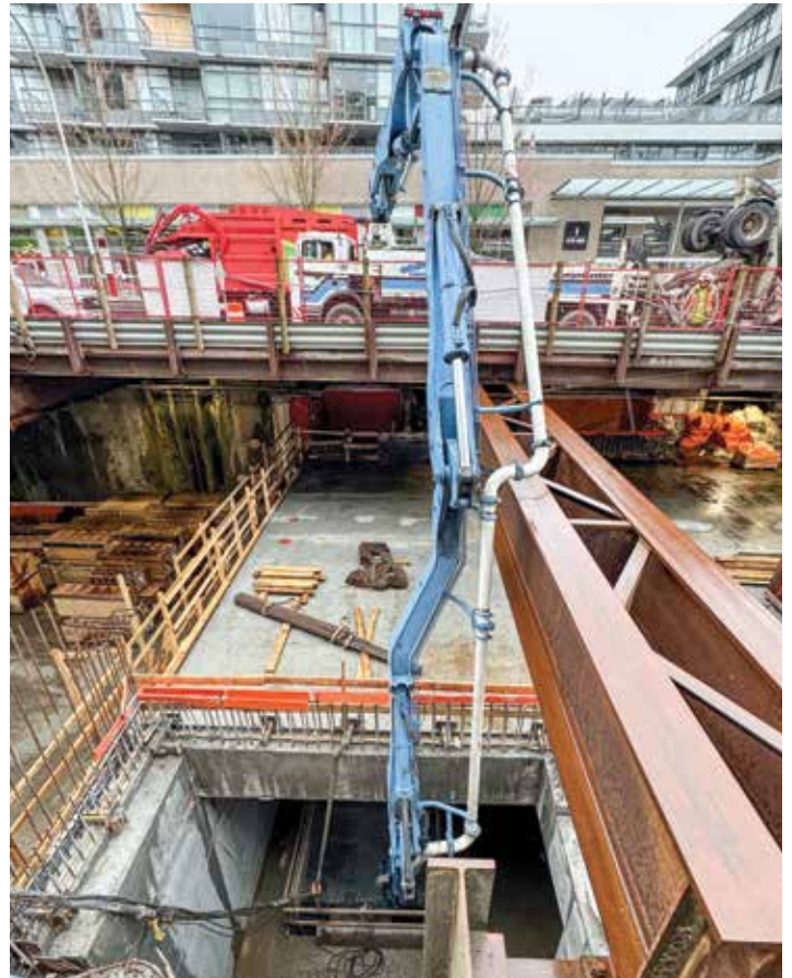
Gastaldo Concrete pumping concrete in tunnel on the Broadway Subway line at Arbutus Street.
