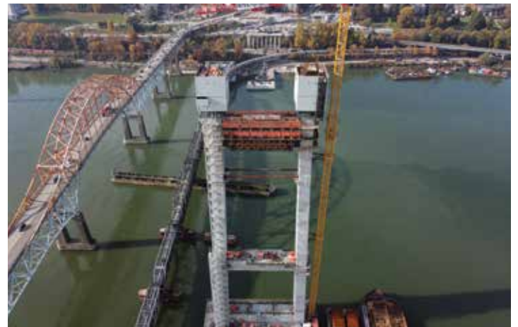
Pattullo Bridge Replacement Project-Main Tower Bridge
