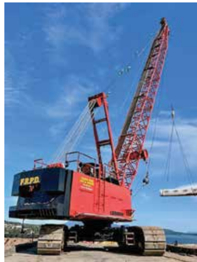
FRPD working at the John Hart Dam Seismic Upgrade Project.
