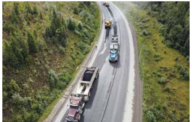
Emil Anderson Construction paving crew in McBride, BC.
