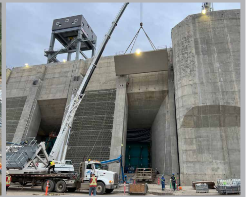
Site C Dam
