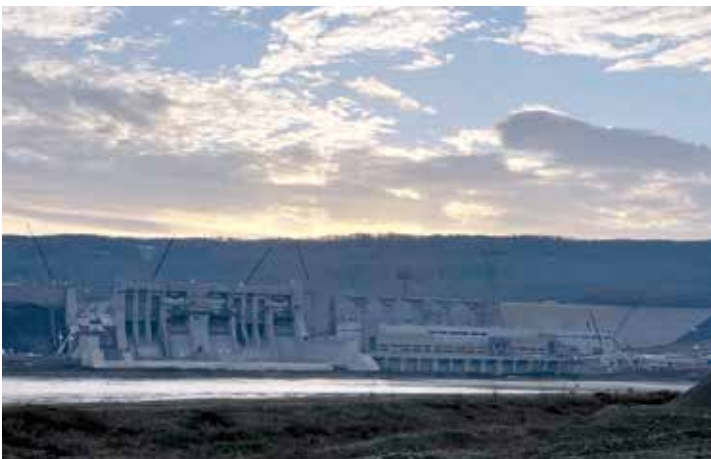
Members working on the Site C dam.
