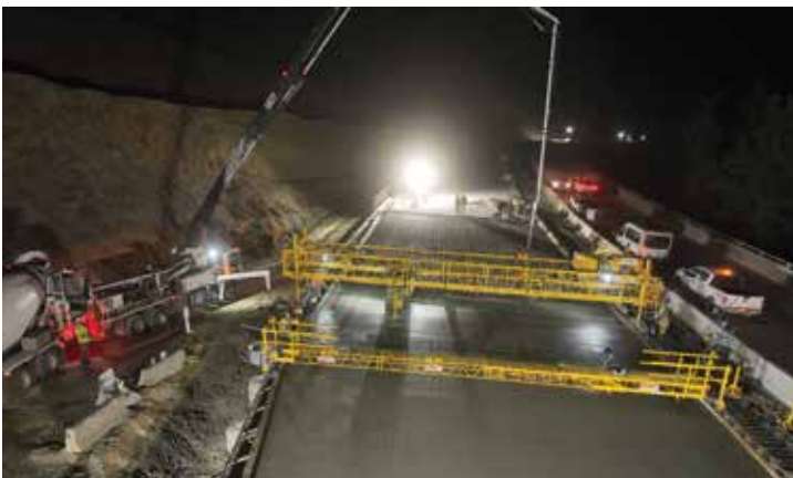
The last deck pour on the Kicking Horse Canyon Project.
