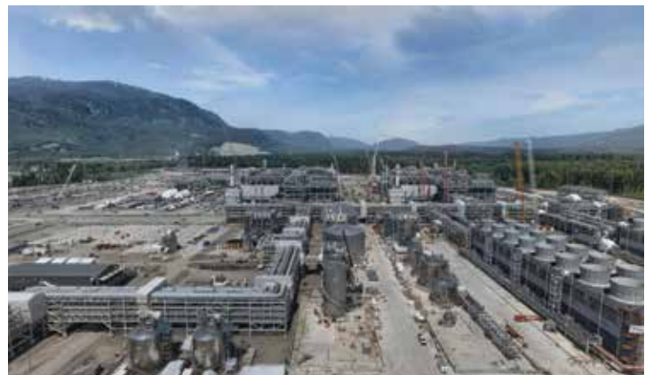
LNG Canada site construction activities, Kitimat, June 2023.
