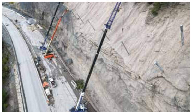
Rockfall protection mesh being installed just east of Dart Creek.
