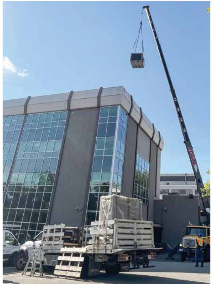
Eagle Crane Inc. doing the heavy lifting to get the new HVAC units onto the roof at the Local 115 Burnaby office.
