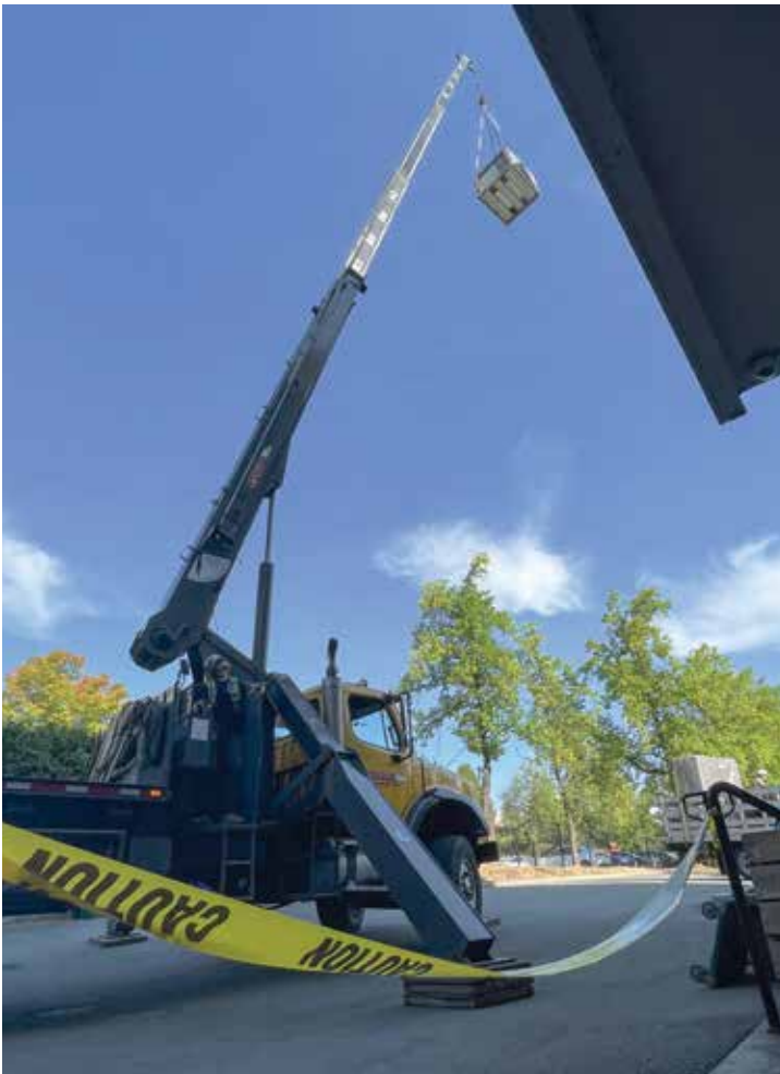
Eagle Crane Inc. doing the heavy lifting to get the new HVAC units onto the roof at the Local 115 Burnaby office.
