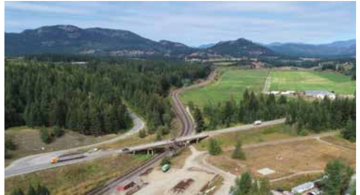
The improvements to the Trans-Canada Highway between Ford Road and Tappen Valley Road was awarded to Emil Anderson Construction.
