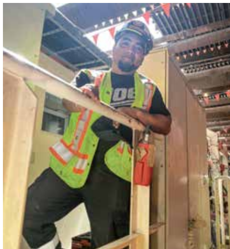
Member Jameson Franco Martinez working at the Broadway Subway Project.
