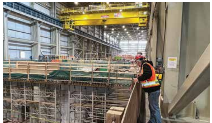
Business Manager Brian Cochrane tours the Site C Dam.
