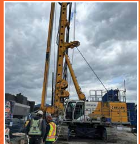
A cutter soil mixer is used to stabilize Keller Foundation's site in Kelowna.
