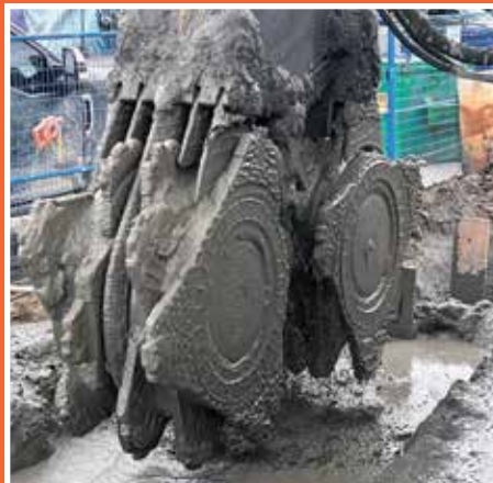
A cutter soil mixer is used to stabilize Keller Foundation's site in Kelowna.
