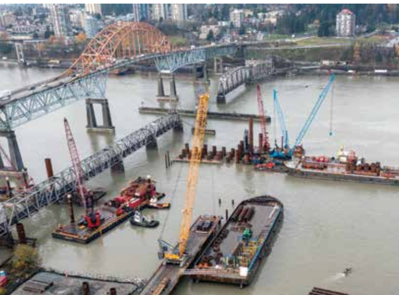
Work on the foundation of the main tower of the Pattullo Bridge replacement.
