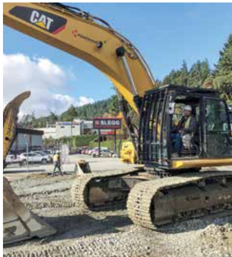
Bruce Korsvoll with Hazelwood Construction.
