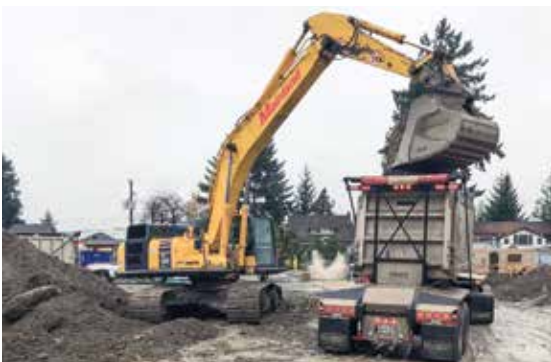
Patrick Sullivan with Mainland Shoring site in Burnaby.
