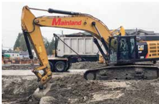
Robert Pavan with Mainland Shoring site in Burnaby.
