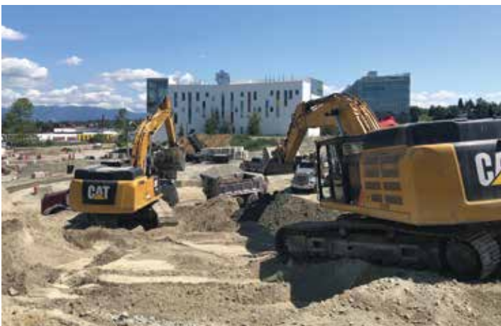
IUOE Local 115 members with Bel Pacific-NorLand Group BC Infrastructure Broadway Project.
