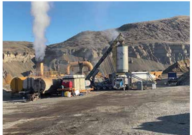
Work in Ashcroft at the Emil Anderson Construction asphalt plant.
