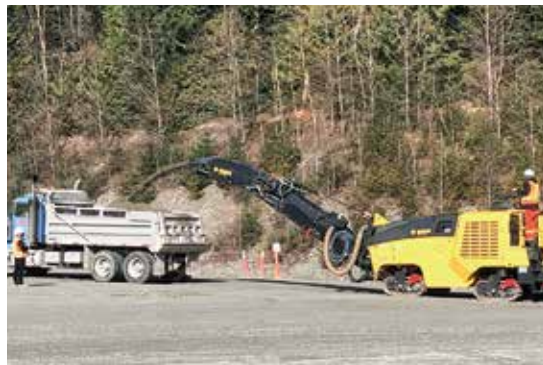
2020 Bomag BM 1200/35 milling machine provided by SMS Equipment for paving courses.
