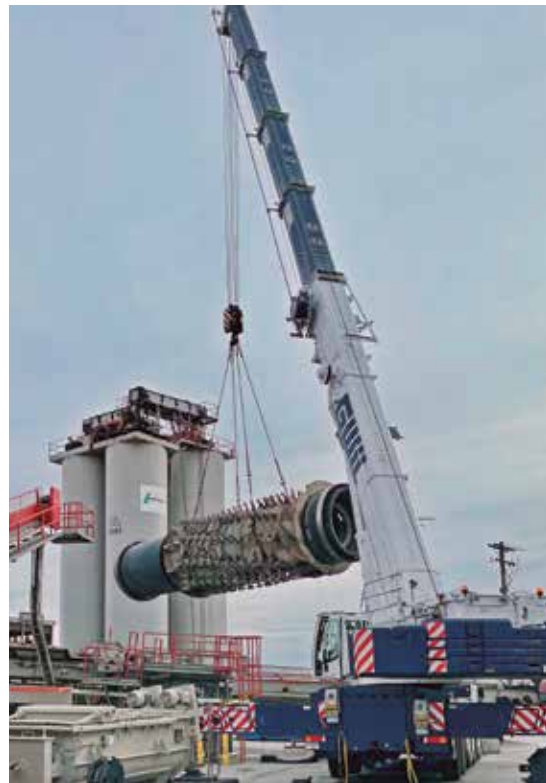
GWIL Crane lifting the main slat out of Lafarge's Port Kells Plant in Surrey.
