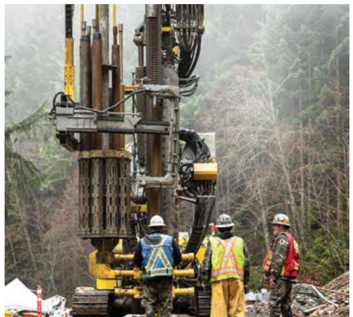
Pacific Ground Engineering's Klemm KR807-7G rock drill on site in North Vancouver, preparing for drilling micropiles at the base of Grouse Mountain *
