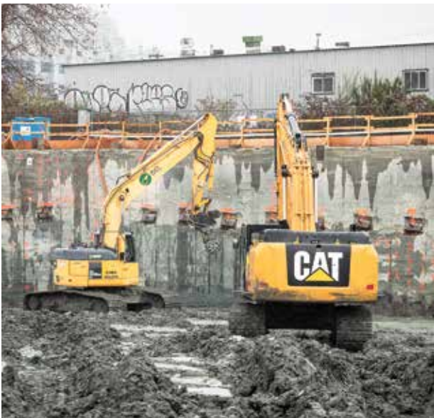
BelPacific Excavating & Shoring crews working on a challenging excavation of approximately 100,000 cubic metres for a new high rise development project in Vancouver
