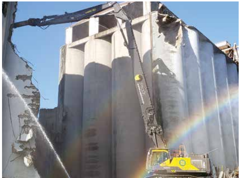
The Pacific Blasting & Demolition crews have been feeling a little lucky on the Viterra Pacific 3 project in Vancouver. Water jets used to suppress dust created quite the rainbow over the new Volvo 480 high reach demolition
