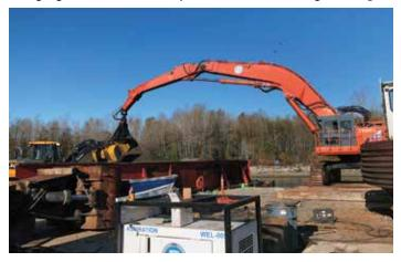
PPM Civil Constructors working on the Maplewood Marine Restoration Project, north shore of the Burrard Inlet in North Vancouver. The general scope of work for this project includes dredging, the infilling of imported sand, fill material to create an intertidal flat and shallow subtidal eelgrass habitats, and the creation of rock dykes and rock reefs.
