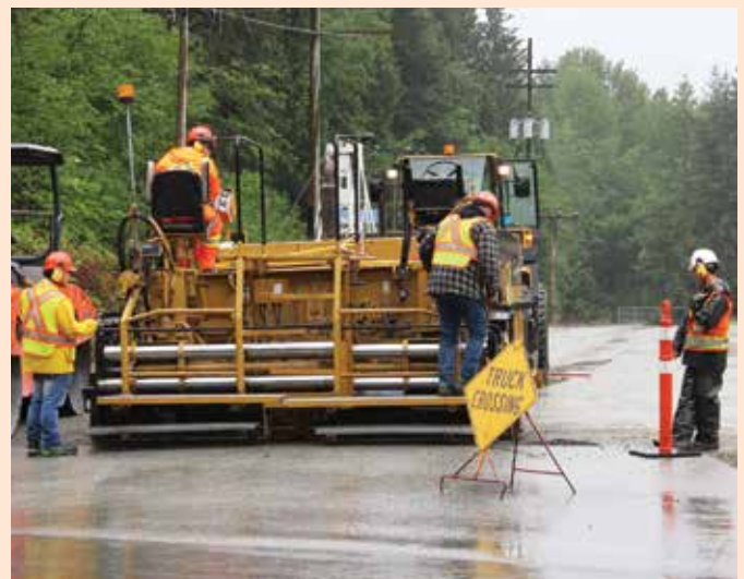
Asphalt Laydown class laying down millings at training site donated by Lafarge
