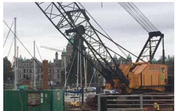
Salish Seas, Victoria Inner Harbour Wharf, 150-ton American, vibro-piling
