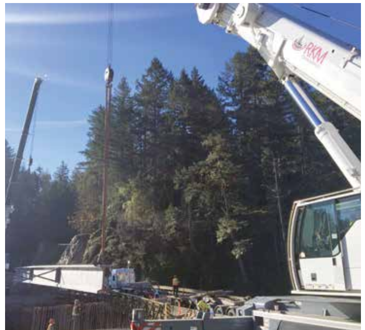
Corrie Thiessen and Bryan Skopnik placing the first concrete I-beam girder. Each crane had 41,000 lbs up at a 75' radius.
