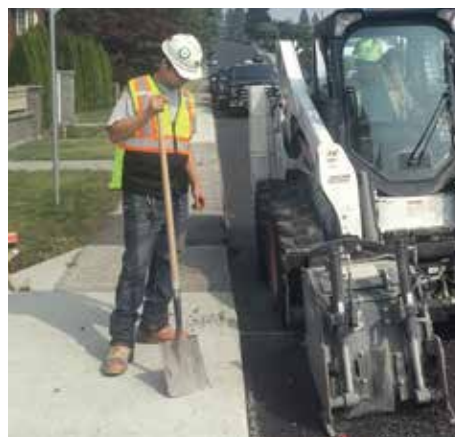
Donald Ducharme running the bobcat and Tony Santos from BA Blacktop grinding for speed bumps in North Vancouver.
