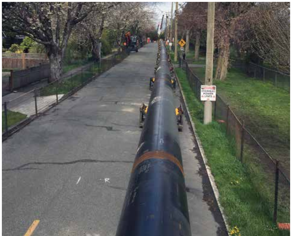
Local 115 District 2 members working with Michels Canada Co. installing 970 metres of a 40" Pipe Main to the new treatment facility on the south end of Victoria. Members working with Advantage Cranes, Gorosh Cranes Ltd. and RKM Crane Services are on site with 6 cranes operating Pre-Roller Support for the Side Booms placing of the almost 1 km of pre-welded pipe.
