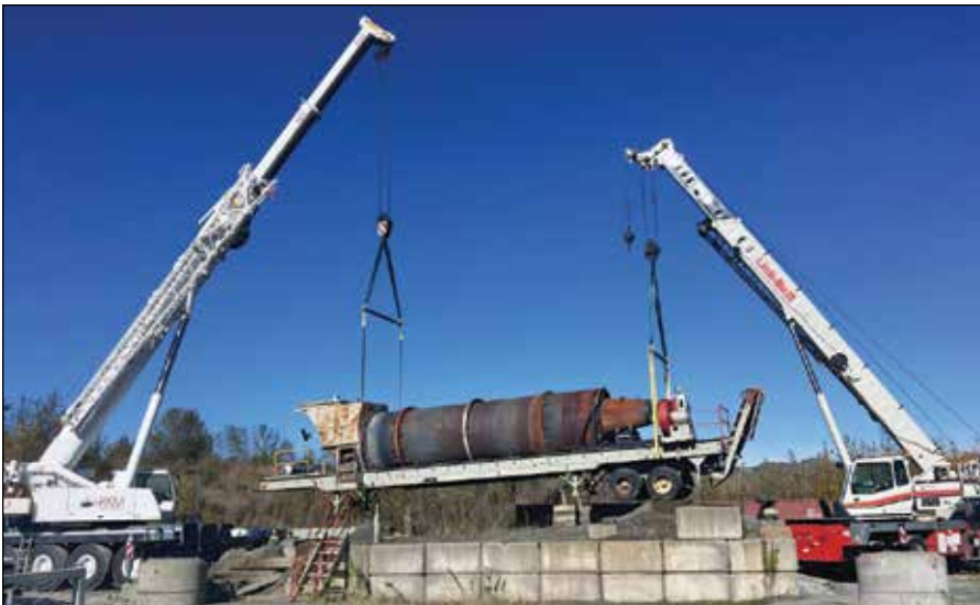
RKM Services Ltd. lifting the drum from the Lafarge Asphalt Plant on Huntingdon Road. Operators L-R: Garret Ewasiuk running the 120 ton crane and Lee Taylor running the 60 ton crane.
