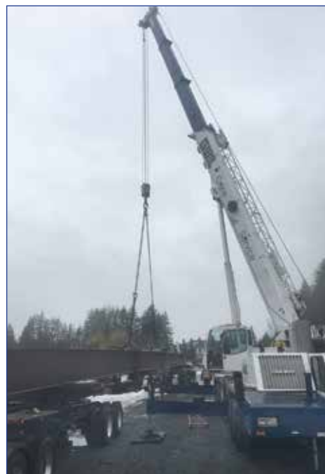
Brother Calvin Meier working for GWIL Crane Service, doing a 40,000lb lift for the Vedder River Crossing Bridge.
