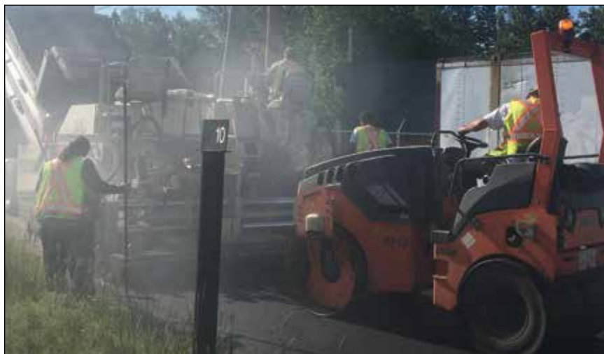
Brother Bert Macdonald running roller behind the Pitman asphalt crew, paving alley ways off of Queensway Street in Prince George.
