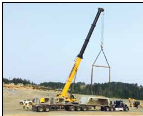
Brother Drew Parsons with Advantage Crane operating a GMK5255 Unloading and placing Pre-Cast Box culvert for Chew excavation at the Royal Bay development.
