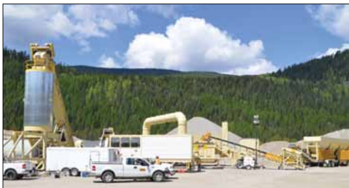
Selkirk Paving Ltd.'s new asphalt plant in Salmo.
