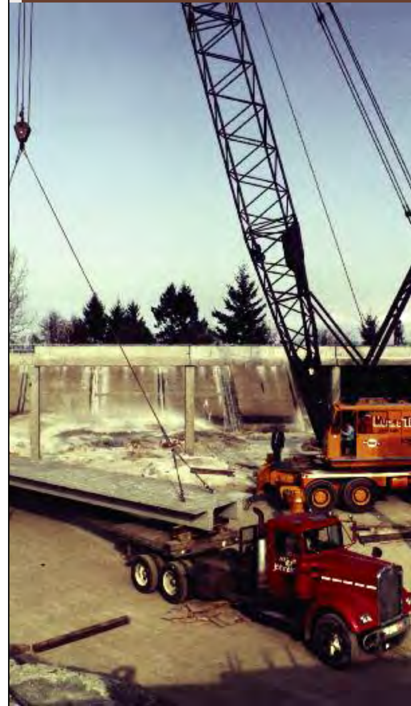
That's a 165-ton American placing a prefab concrete slab on a truck bound for the Broadmead Water Reservoir in Victoria in April of 1982.
