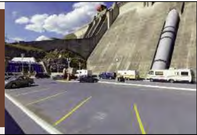
A giant whirley crane is fitted together in this aerial view of the Revelstoke Dam under construction (left) in 1979. Six years later the cement dam rose 175 metres high (right) to provide the capacity to generate electric power and also to control the Columbia River to present flooding.
