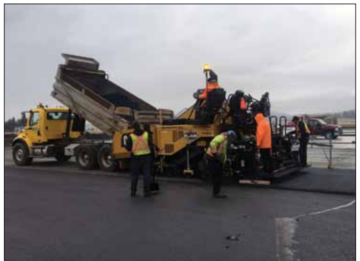
Island Asphalt crew working at the Victoria airport.
